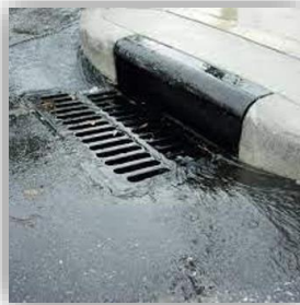
Storm Water Drains
