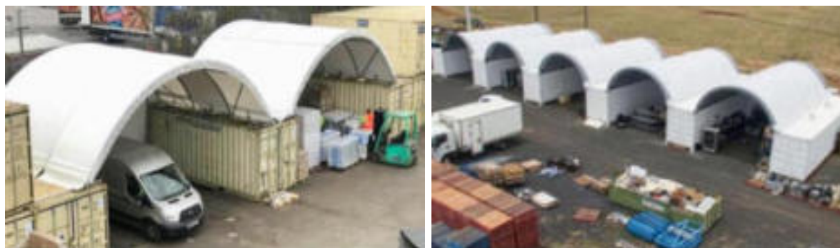
Figure 12: Example of how multiple shipping containers and canopies can be combined to establish larger partitioned and organised storage
