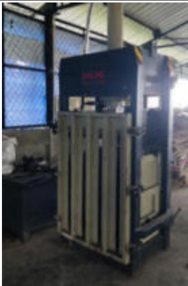
Baling Unit at SLRM center Source: Consultant team (field visit)
