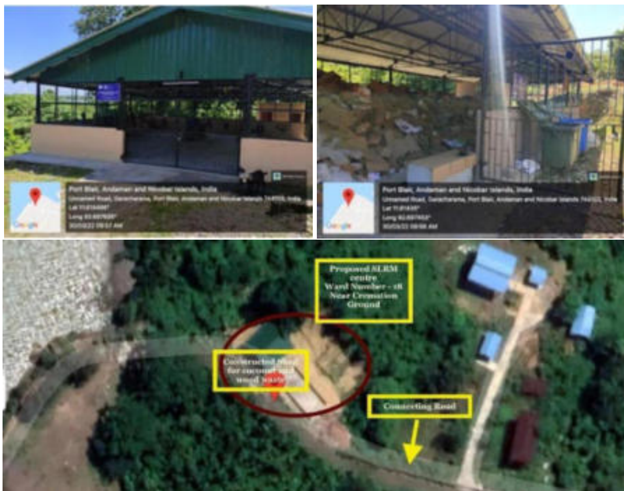
Figure 8: Garacharma SLRM location, dry waste processing (left), wet waste composting (Right). (Google Earth)
